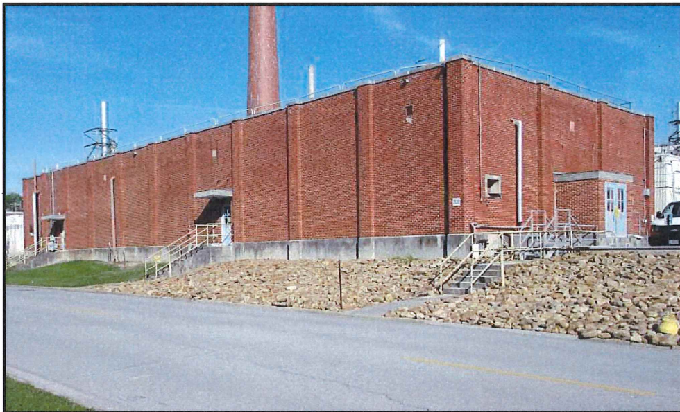
Figure 9. Overview of east and south elevations of Building 3038.
