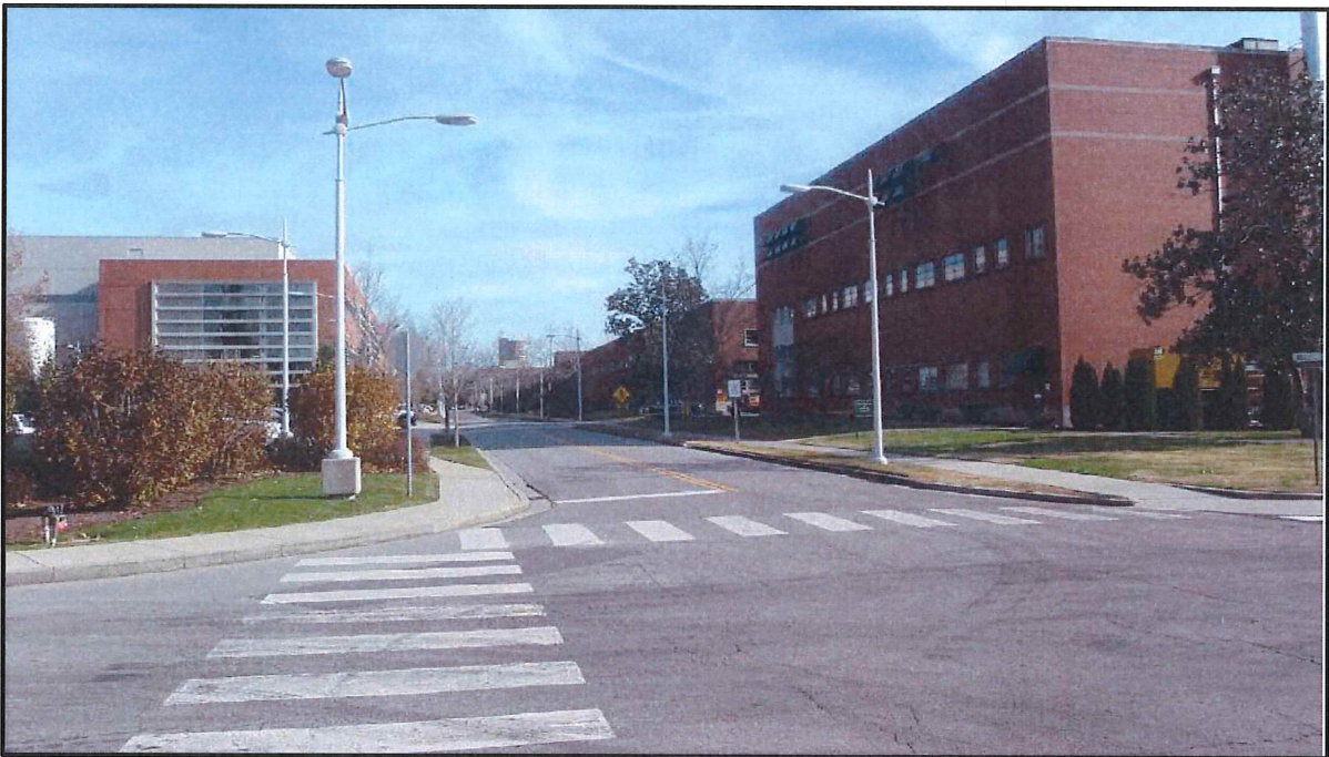
Figure 15. View east along Central Avenue showing Buildings 4501 and 4500N (right) and 4100 (left).
