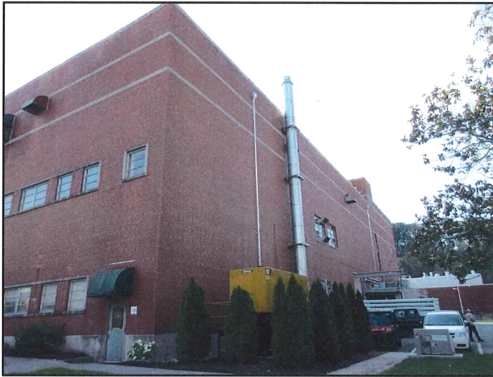
Figure 12. West elevation of Building 4501.
