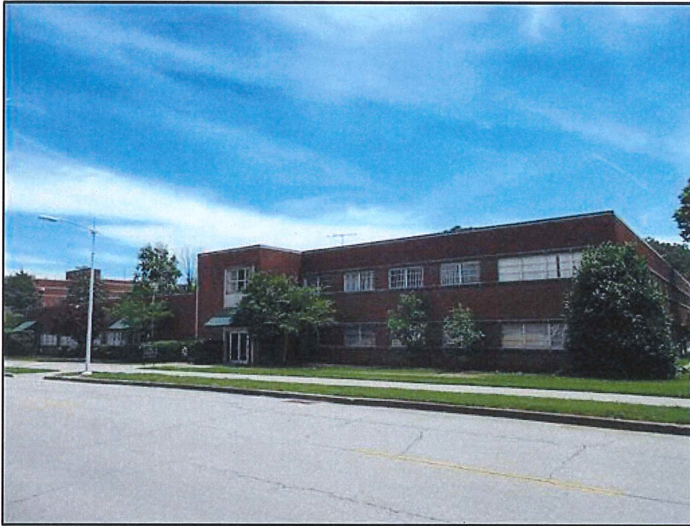
Figure 6. Overview of the façade of both sections of Building 3500.
