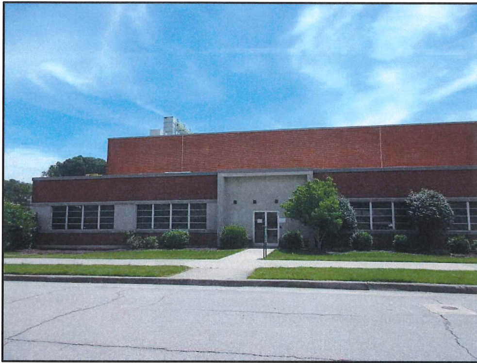
Figure 7. Overview of north elevation of Building 3525.
