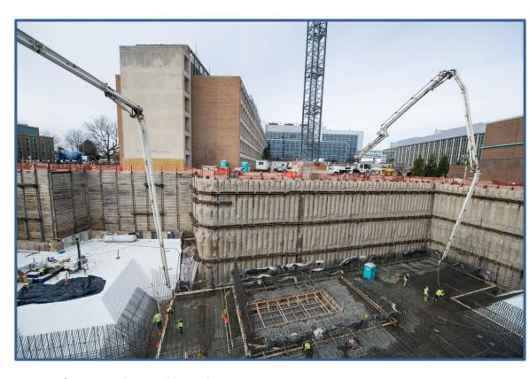
Concrete for the floor of the target area was placed December 1-2. It took around 30 hours and 300 concrete trucks to place the 2,700 cubic yards of concrete. FRIB received Critical Decision 3B, Approval to Start Technical Construction, on August 26, 2014.
