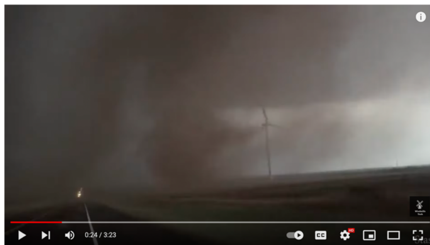
Figure 13: Extreme Conditions: Can Wind Turbines Survive Tornadoes Wind Speeds
