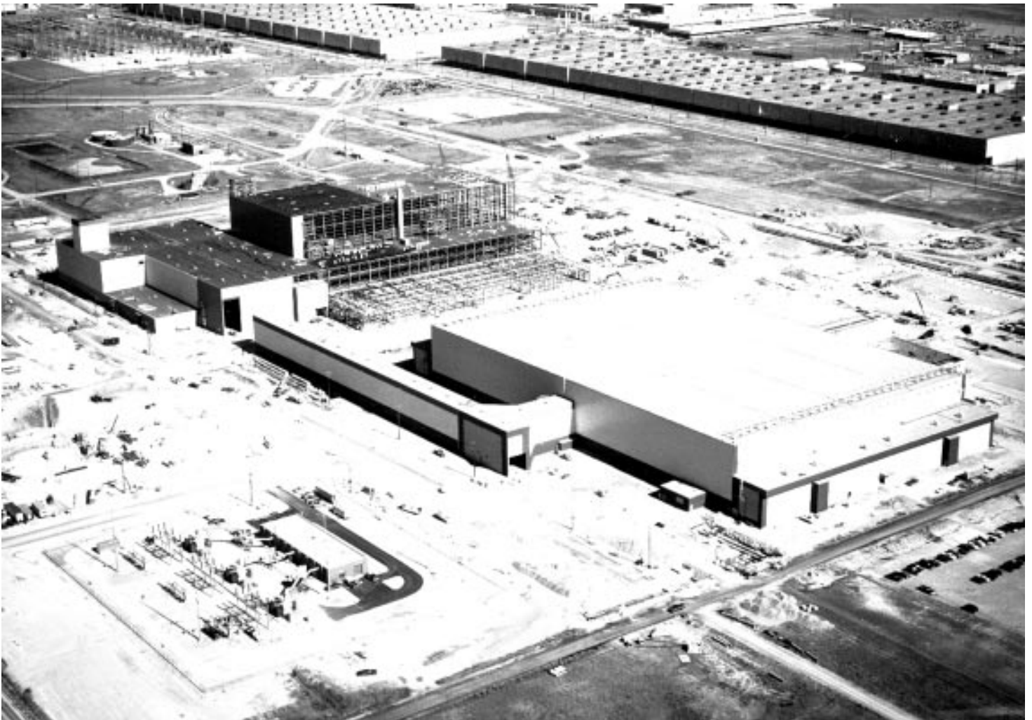
Figure 2.1: Gas Centrifuge Enrichment Plant
