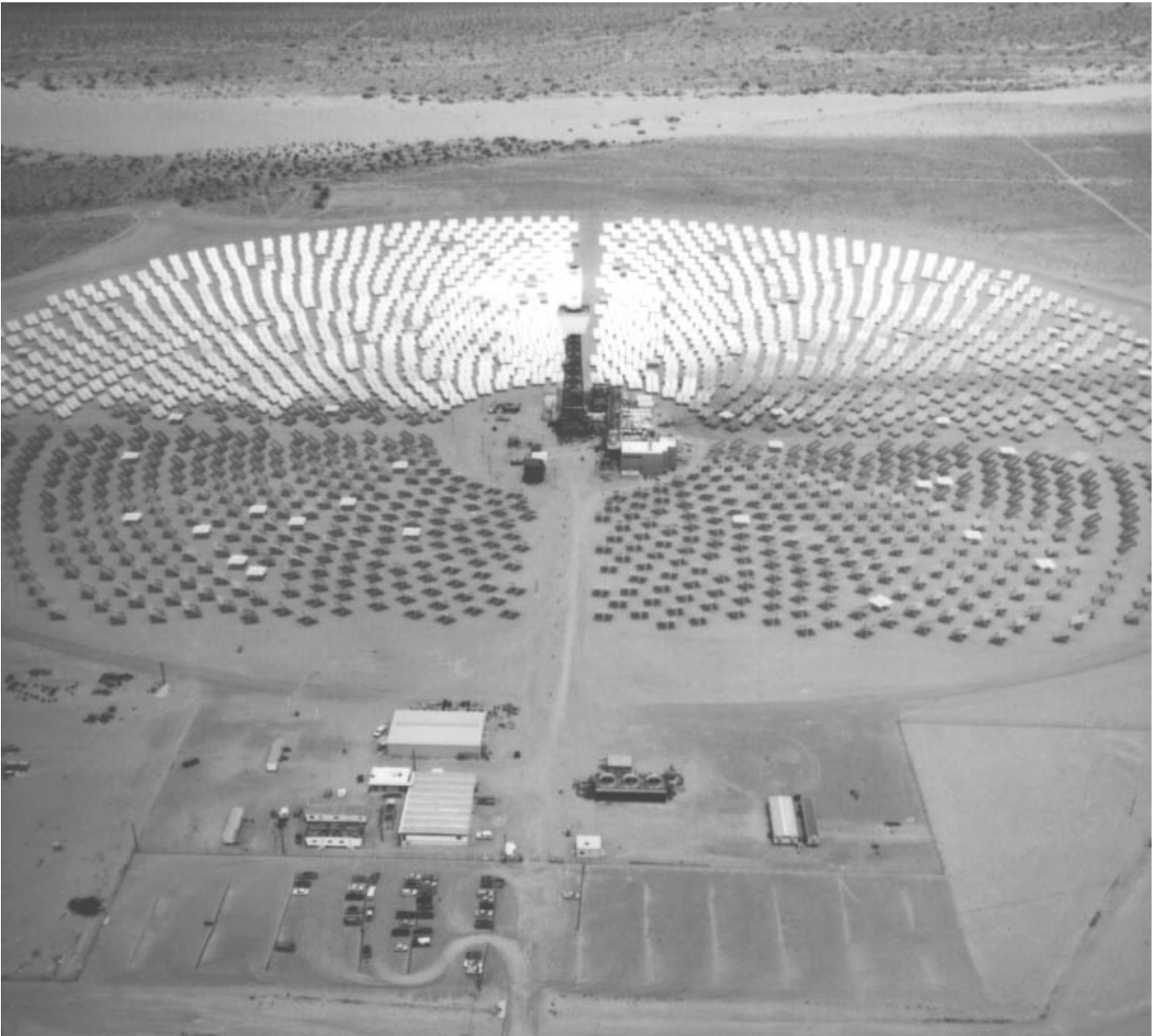
Figure 1.4: Central Receiver Solar Thermal Power Plant
