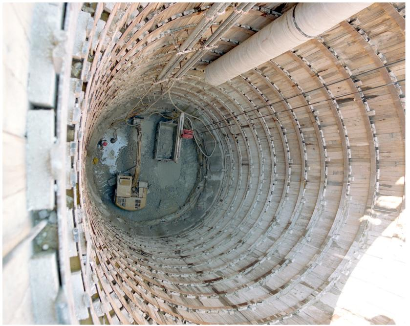
The decay tunnel as excavated by the Tunnel Boring Machine (TBM). TBM is far in the background.
