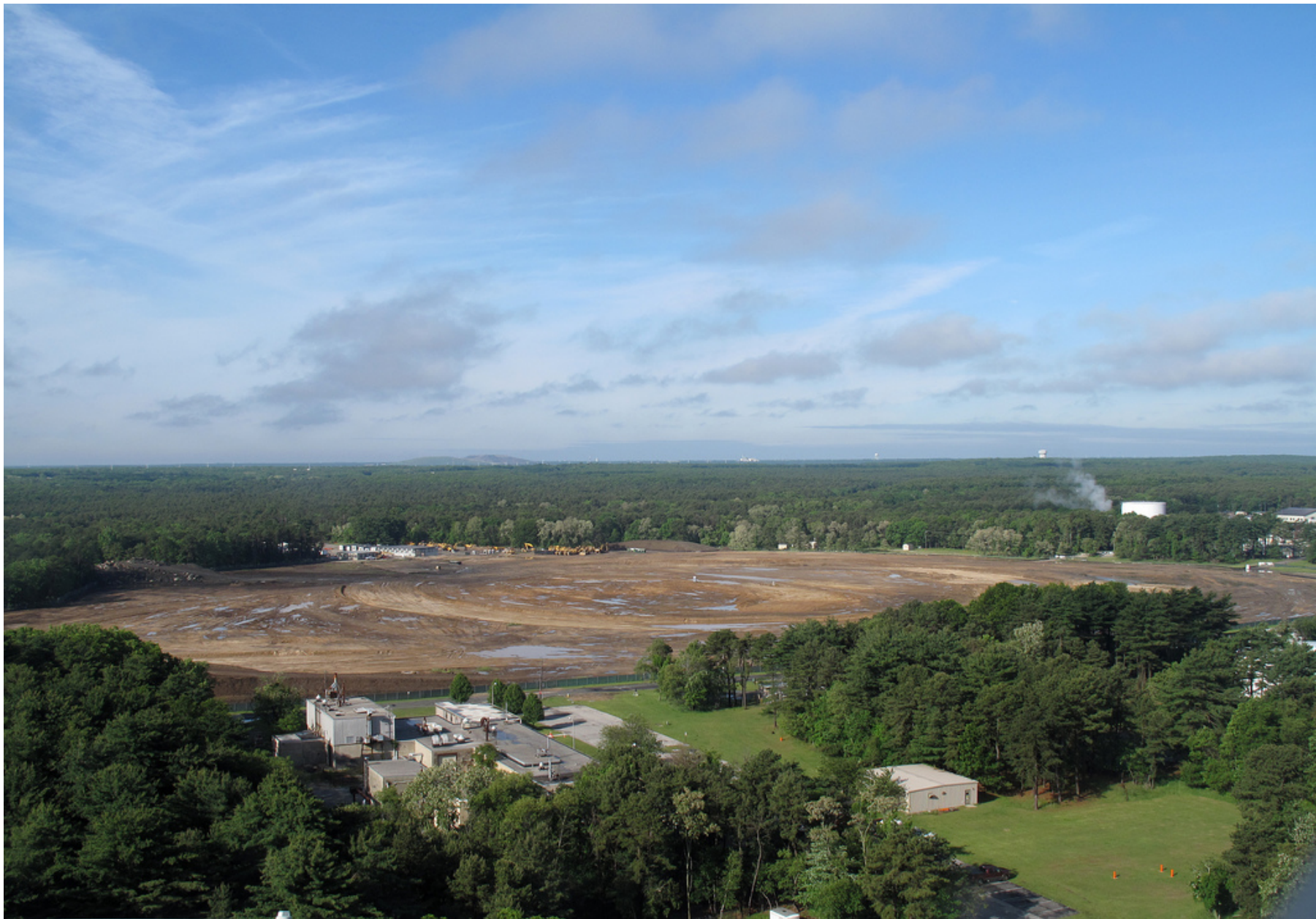
Construction site of the National Synchrotron Light Source II on June 6, 2009
