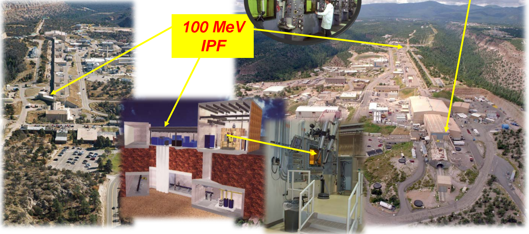
LANSCE Accelerator Complex
