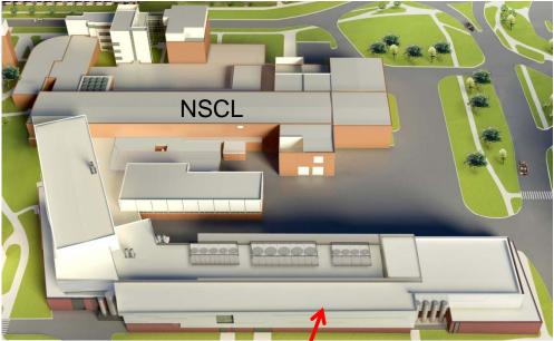
New FRIB Linear Accelerator Front End Tunnel is ■ 550 ft long **7**0 ft wide **Beam Delivery** 25 ft underground
