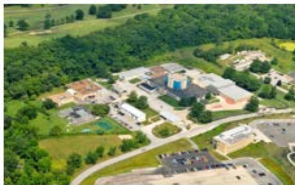
Figure 1. General layout of the MURR facilities
