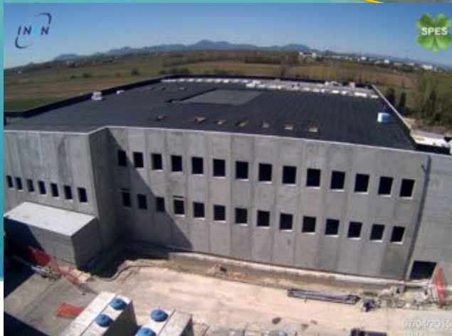
RIB Beams in 2018-19
