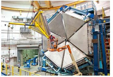
Mounting of the Forward Time-of-Flight detector arrays onto the forward carriage in Hall B Project was re-baselined in September 2013 with a Total Project Cost of \$338M and completion in September 2017
