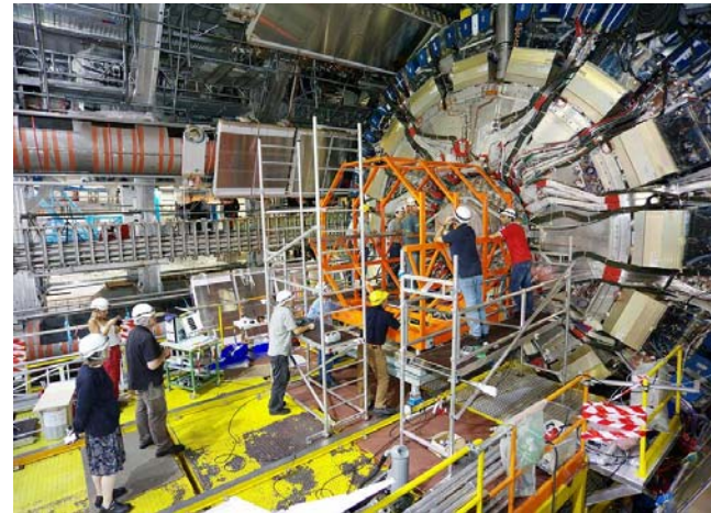
8/24/06 Barrel inner detector (SCT & TRT) being inserted in the bore of the Barrel Calorimeter
