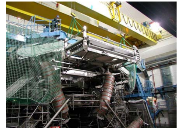
Barrel Muon station being installed
