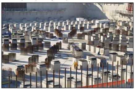
Precise and careful alignment for Seismic Pad #100: Early November 2011, workers completed the installation of seismic pad number 100.
