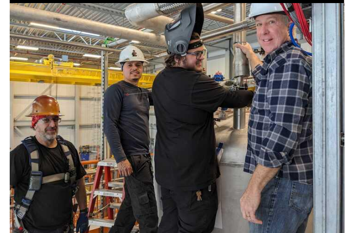
Dec 1, 2023 welding last cryogenics line
