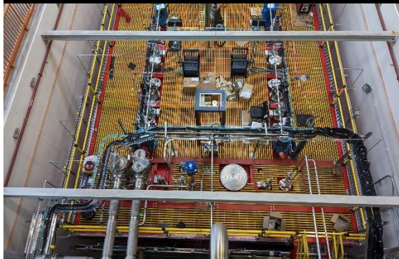
October: Cable Routing Complete
