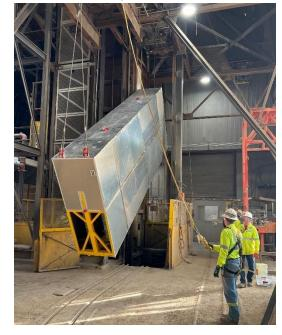
Shipping container, holding two APAs, is moved into the Ross Shaft at SURF to be lowered to the 4850L
