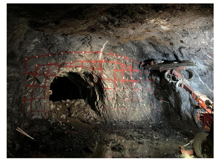
Drilling Charge Holes in the 4850-81 Face
