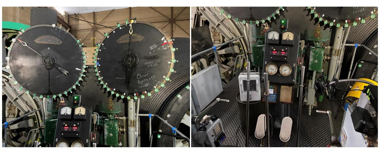
1930-era Control System - Foot Pedals, Analog Gauges, and Hand Levers - replaced with state-of-the-art digital control system
