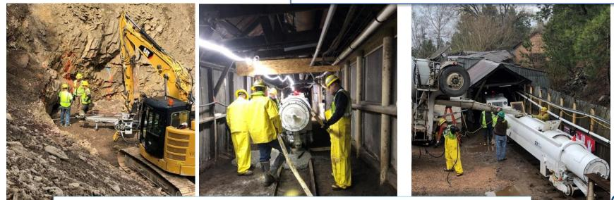
Refurbishing the 2400' long tramway that the 4100' rock conveyor will be installed in to move rock to the open cut in downtown Lead, SD
