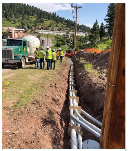
Rerouting power underground so elevated conveyor can cross state highway
