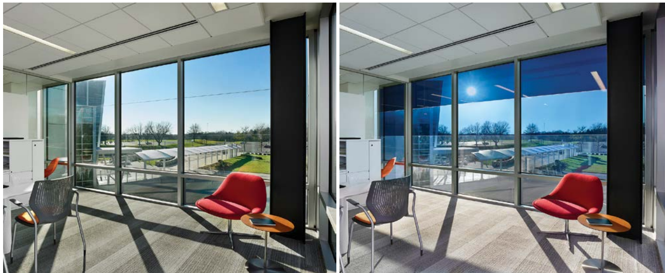
These “smart” windows make use of specialized materials to change their tint and lower the amount of sunlight transmitted in response to environmental conditions, saving energy for cooling buildings and creating more comfortable working conditions. ( SageGlass, Inc )
