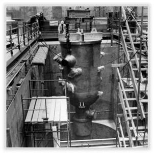
The HFIR pressure vessel built by the former Allis-Chalmers Manufacturing Company was installed in April 1964 and has continued to operate reliably for more than 55 years.
