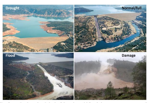
Photos illustrating the wide range of water levels at Oroville Dam and associated challenges faced in managing water in an environment of extremes, for which variability is driven by atmospheric rivers.
