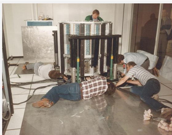
Figure X: Staff at the National Magnetic Fusion Energy Computer Center install a Cray-2 machine.
